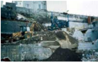
The Gallery in construction
