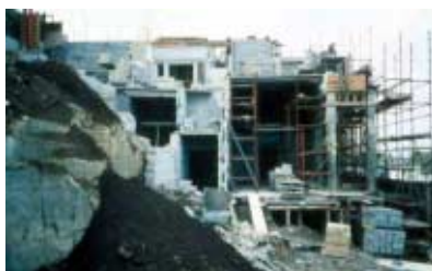
Tate St Ives in construction
