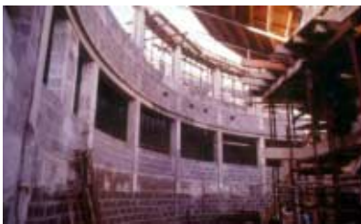
The Gallery in construction
