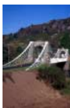
Dredge Suspension Bridge, Great Glen
